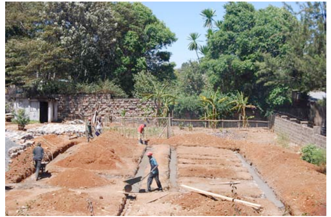
The foundation is poured...by hand
